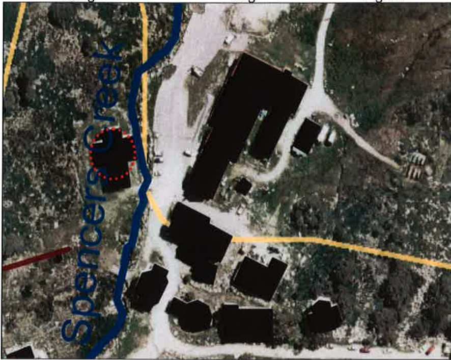
Figure 3: Aerial photo of the location of Bellavista staff accommodation building
